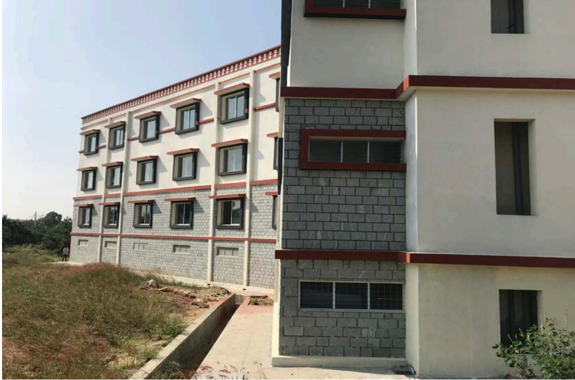
View of classroom block II from the east
