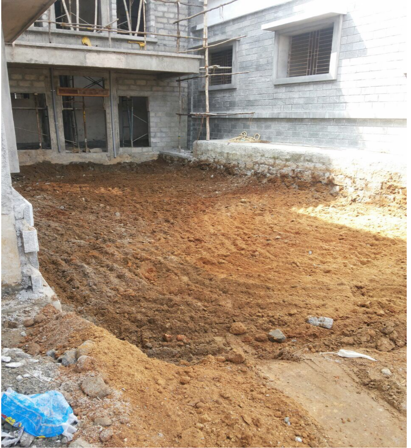
Excavation started from the main entrance of the Boy's Hostel II
