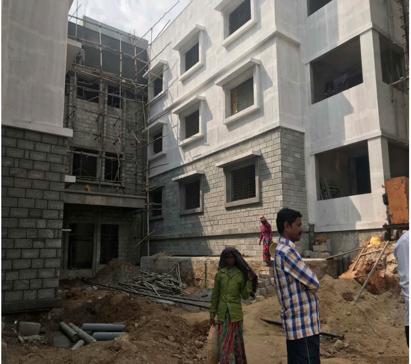
Only portioned remained to be plastered (BOY'S HOSTEL II)
