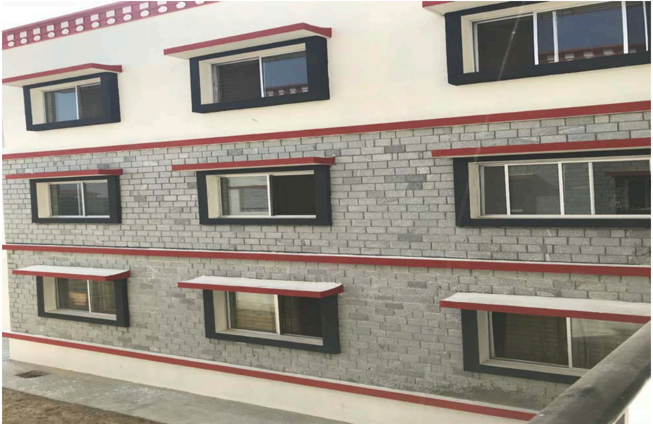
Showing stone cladding work on Hostel Block II
