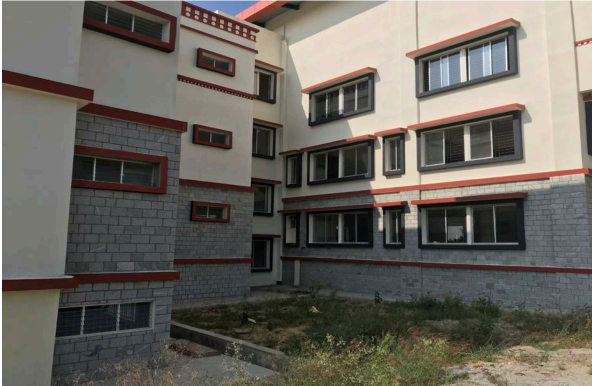
Stone cladding work completed at the back of classroom block II
