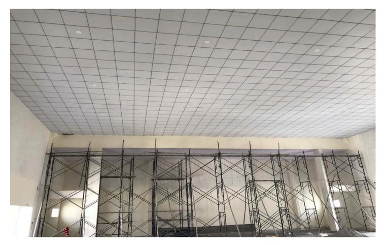
PVC false ceiling with LED lights and side walls being plastered
